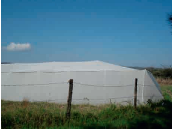
Figure 10. Pavilion in the State of Chiapas (source SIAP).
