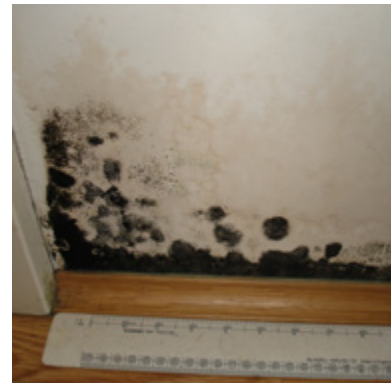
Flooding can cause potentially harmful fungi to thrive on the interior walls of buildings (photo: G. Godwin-Keene)
