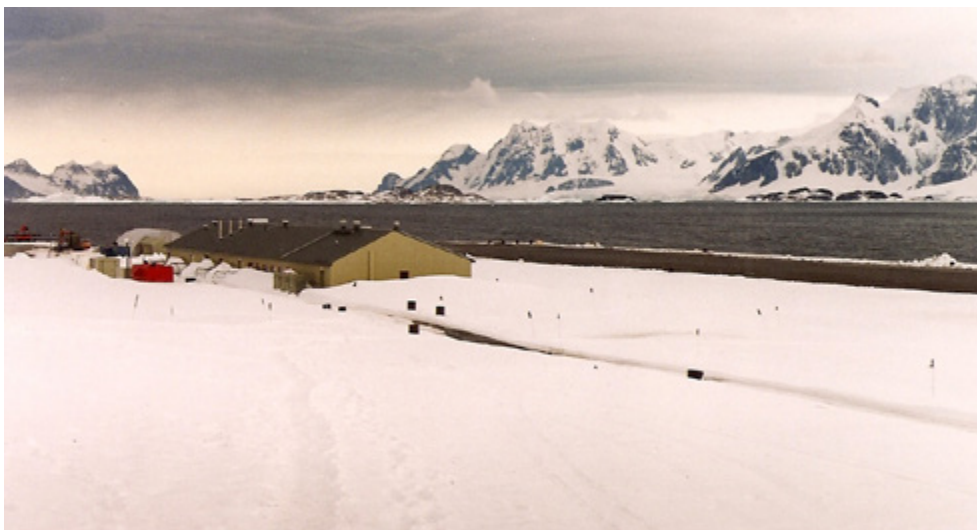
Biology laboratory, British Antarctic Survey, Rothera Research Station, Adelaide Island (photo: P. Bridge)
