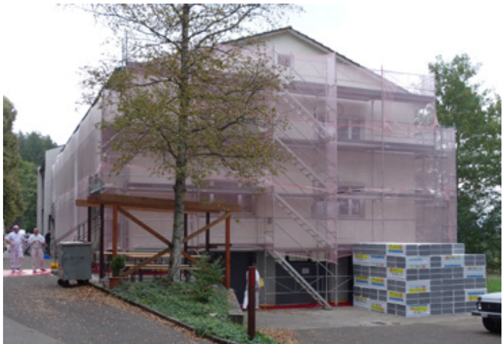
West side of the CABI building, 12 September 2014 (photo: A. Gassmann)
