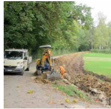
Digging a trench for the fibre-optic cable (photo: A. Gassmann)
