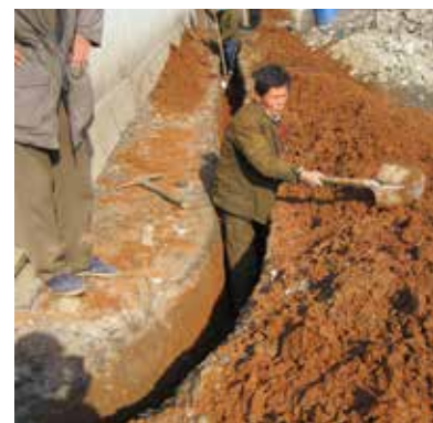
Staff of the Crop Cultivation Institute, AAS, laying fibre-optic cable (photo: Chae C.S., AAS)
